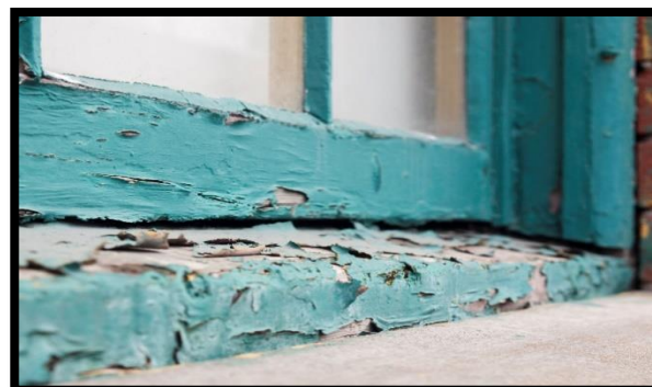
Lead covered porch column and windowsill
