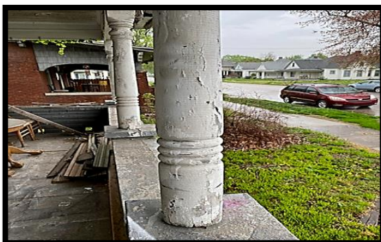
Lead covered porch column and windowsill
