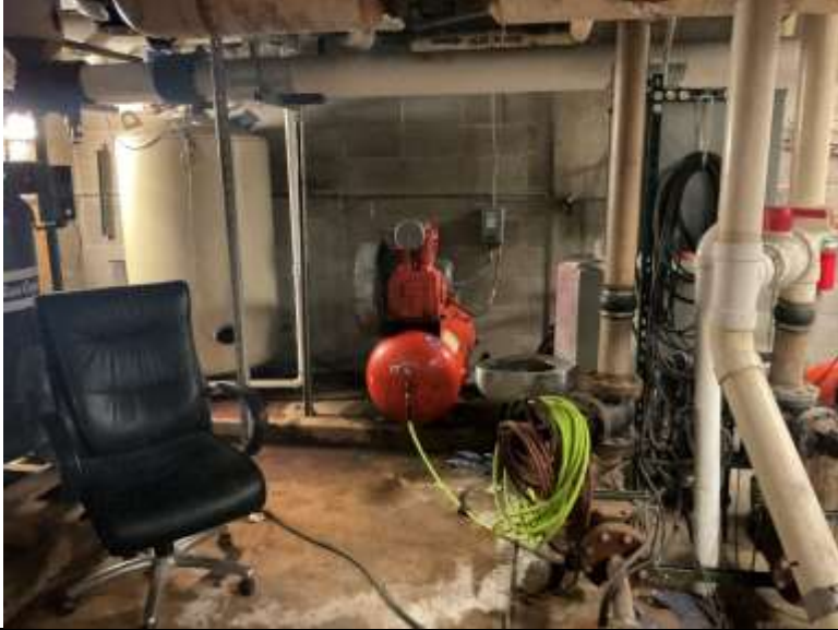
Photo 5: Air Compressor used for pneumatic controls in basement.
