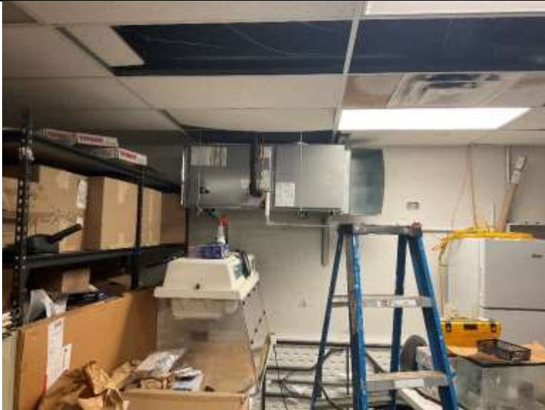
Photo 6: HVAC Unit serving the room with the security electronics equipment. Unit in good condition.
