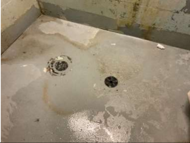
Photo 13: 2000 Renovation Housing Unit. Floor drains in shower in poor condition.
