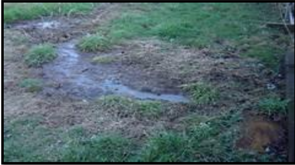
Failing Septic System
